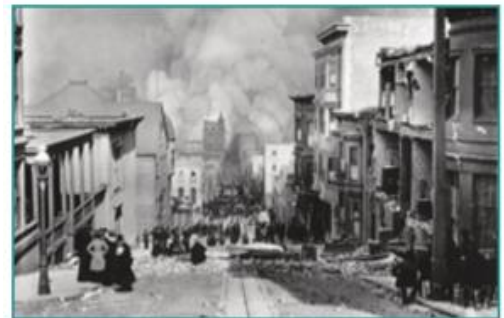
San Francisco Earthquake 1906
